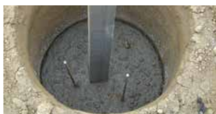
Piedi da cementare Feet to be fixed with concrete
