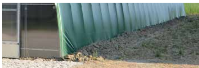
Telo interrato Sheeting to be buried
