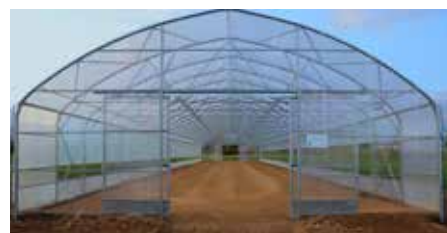
Testate in polycarbonato con porta scorrevole Polycarbonate gables with sliding door
