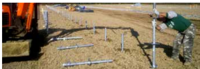
Piedi da avvitare Feet to be screwed into the ground
