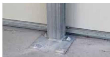
Piedi da tassellare Feet with chemical dowels
