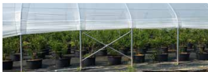
Telo laterale da alzare manualmente Side sheeting to be lifted up manually
