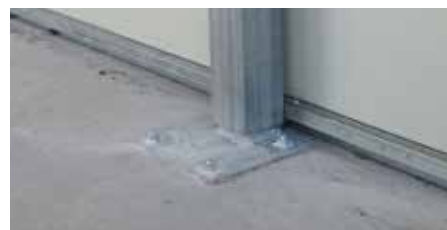
Piedi da tassellare Feet with chemical dowels
